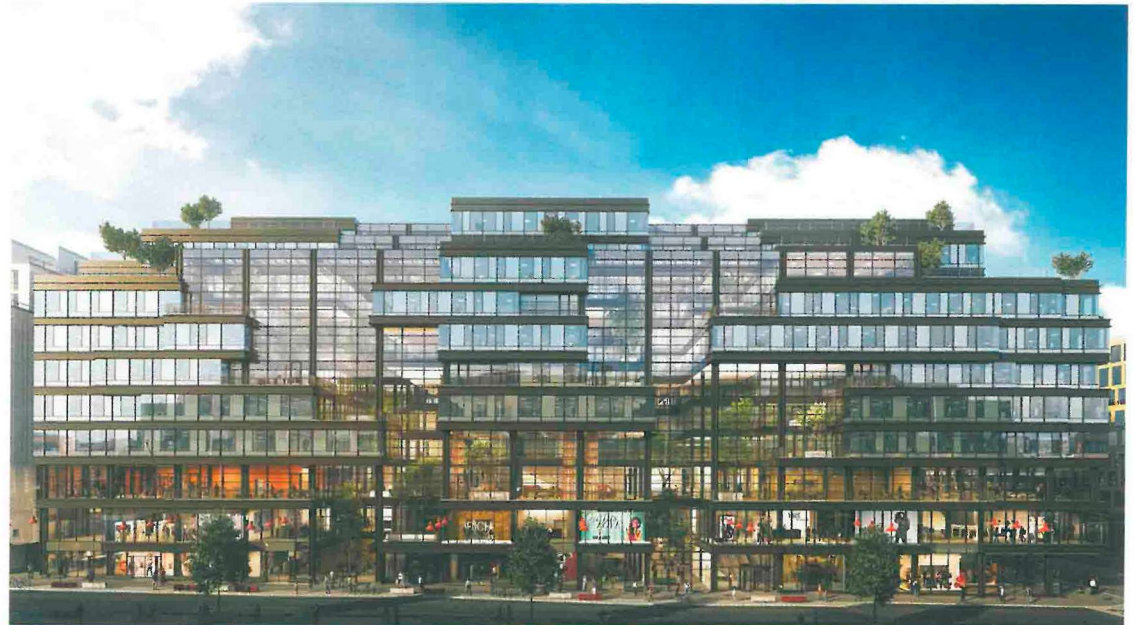
Urban outfitters: AMF is substantially through refurbishment of Gallerian, Stockholm.
