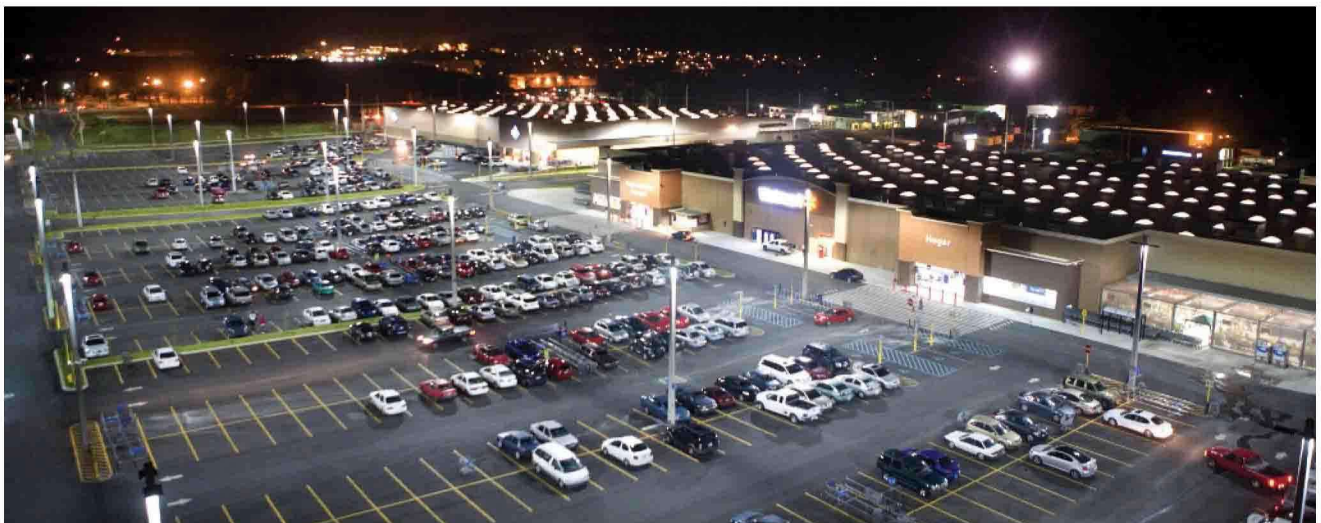
▲ Walmart parking lots are a lot brighter thanks to a massive lighting project that saved millions and improved the customer experience.
